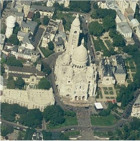
Sacre Coeur, constructed 1875-1914 Paris
